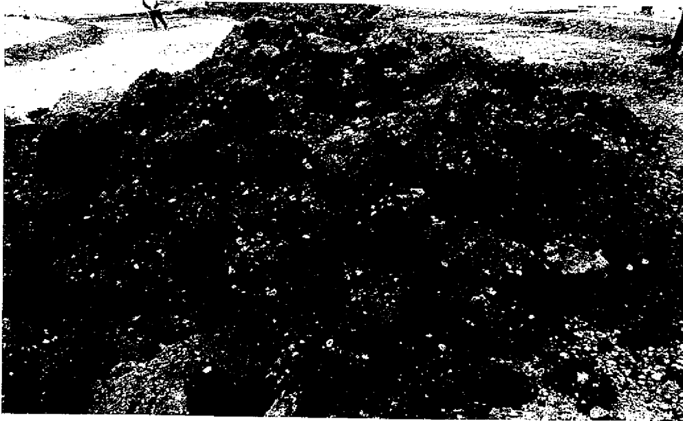
Figure 5 “6F2” material stockpile during removal
